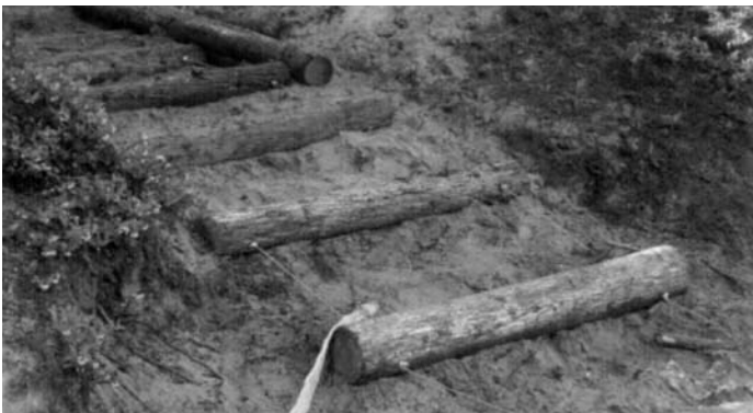
Steps being positioned
