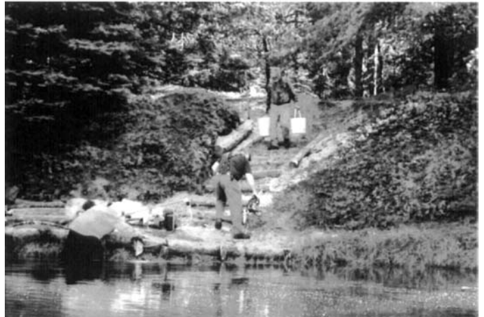
Footer being finished
