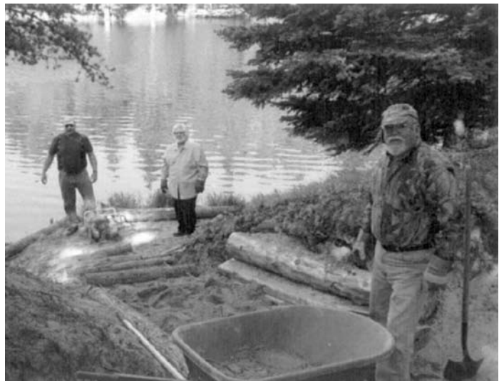
Workers setting steps in place
